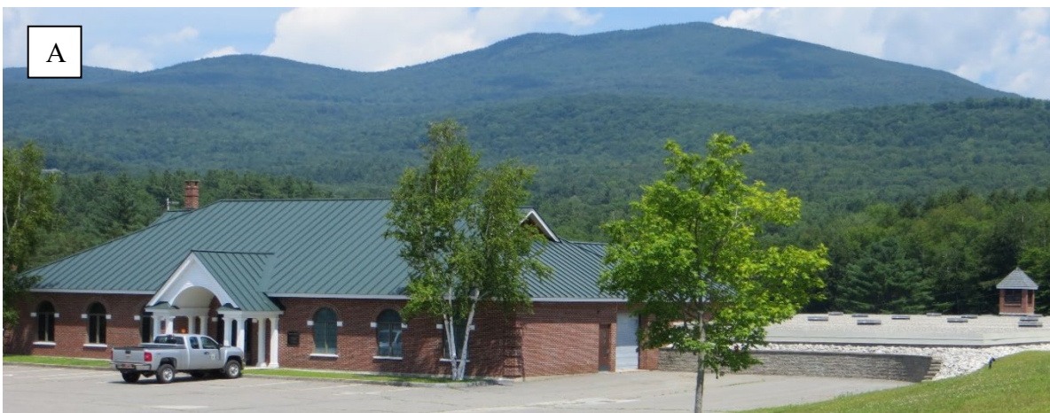
A) 3.6 million gallon per day, slow sand water filtration facility
